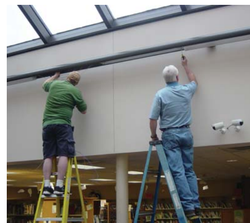
Brian Harvey and Jon Beck replace ballasts and bulbs at the Indianola Public Library
